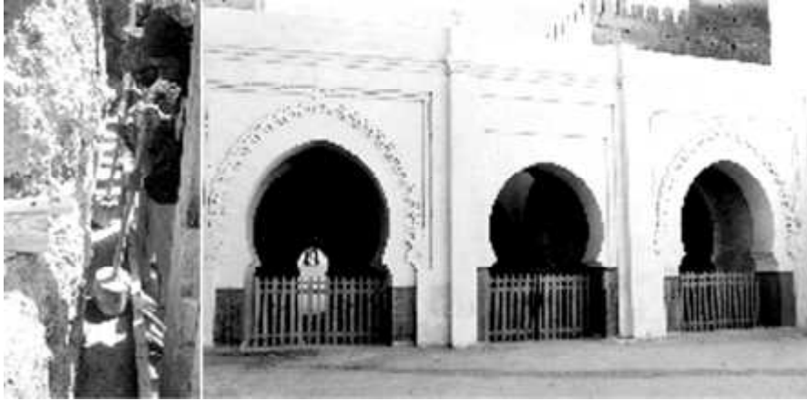
Figure 23.4 Restoration of historic walls
